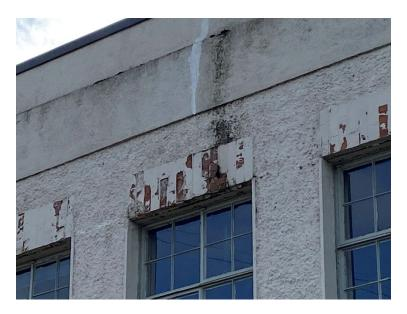
Figure 22: Detail of cracking above first floor windows on north façade
