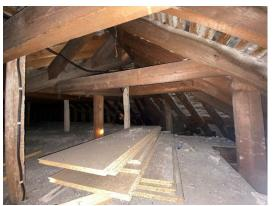
Figure 61: Each cut rafter retains a collar at high level
