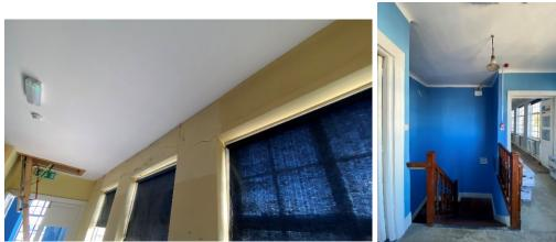
Figure 55: Replacement plasterboard ceiling at first floor level with folding attic stair access
