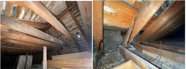
Figure 59: Roof configuration of evenly spaced cut rafters supporting closely spaced slating battens with mortar parging between them, most of which has fallen to the attic floor
