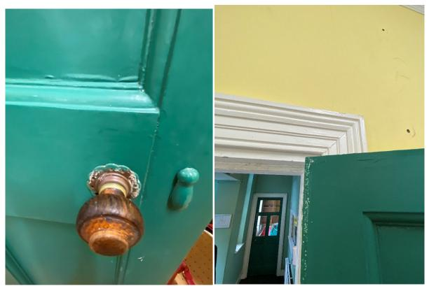
Figure 42:Original ironmongery, likely to have come from a catalogue rather than a bespoke design for the building Figure 43: Typical moulded architrave and panel door details
