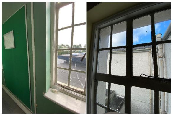
Figure 49: Detail of steel window sitting in timber sub frame Figure 50: Detail of pin stay mechanism
