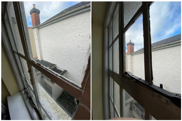
Figure 51:Windows have T-bar sections; all astragals overlap rather than a splice joint.
