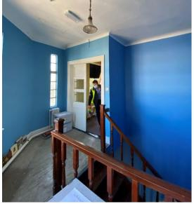
Figure 57: Plaster damage due to water ingress to ceilings at first floor level and above window heads. Note oak floor Figure 58: Main staircase with unusually widely spaced spindles
