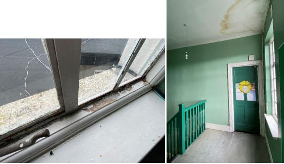
Figure 46: Detail of steel windows which are housed in timber moulded sub-frames with timber window boards
