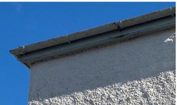
Figure 72: Roughcast plaster harling and brick
