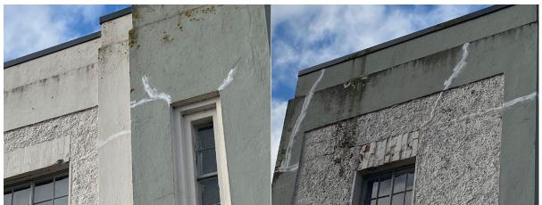
Figure 26: Cracks above windows on Eastern façade
