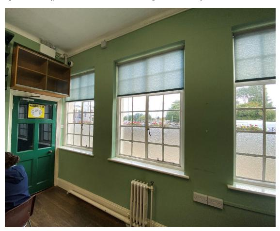
Figure 41:Original library reading room, with simple coved cornice, panelled doors, moulded architraves, cat-iron radiators with surface-run pipework. Smooth plaster walls with paint finish.
