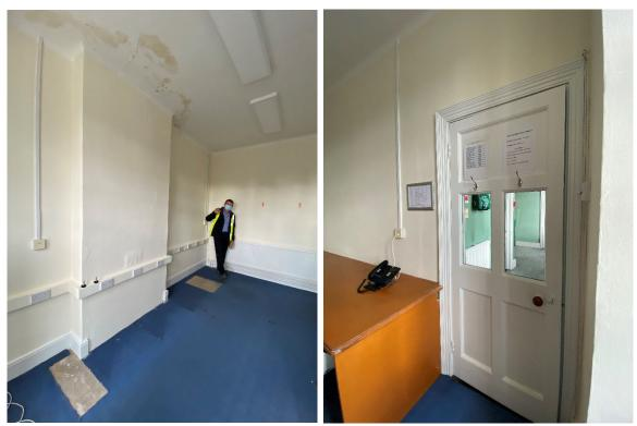
Figure 47: Evidence of significant water ingress around chimney breast at first floor level.
